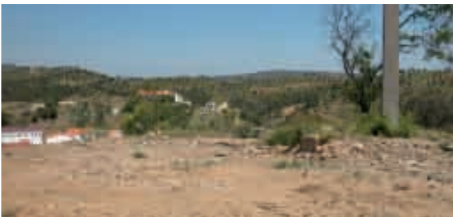
Terraplanagens na nova Ze2
